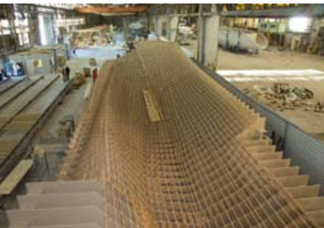
Photo Drassm, S. Cavillon
